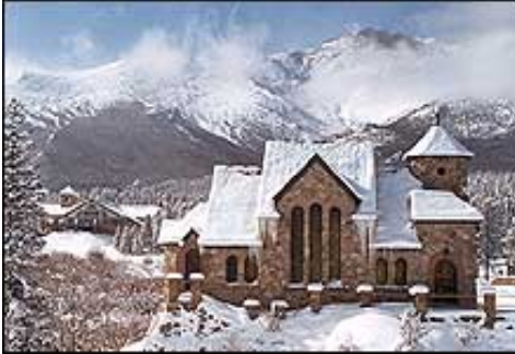
St. Malo Retreat Center Stanley Hotel Estes Park, Colorado
